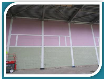
Within the sports hall the process is the same. Below the plasterboard is a fire lining board. All of these need to be cut to fit the steel sections. These will shortly been tape and jointed and then painted to design.
