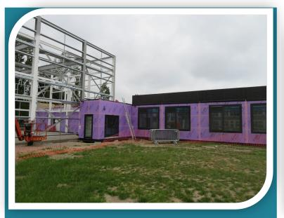
On top of the modules a parapet has been installed to provide a edge protection for operatives that undergo maintenance on the roof. It also acts as a barrier with the services on top of the roof and pedestrians below.
