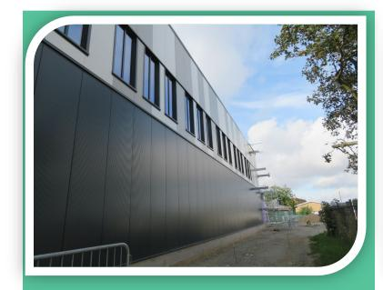
The sports hall is traditionally built. At Clacton the steel frame requires cladding. This cladding is an insulated panel and fixed to the steel frame.
