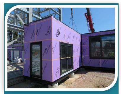
In this project there was a total of 22 modules that were delivered and then lowered into place using a 350tonne crane. The installation team had to plan the lifts and secure the modules into place.
