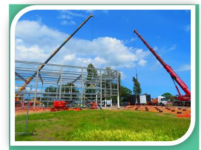
The steel frame is installed using a team of steel fixers and crane drivers. This structure is the skeleton of the sports hall which then receives external cladding and block and beam floor system.
