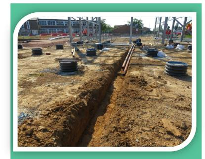
Under slab drainage needs to be installed before the modular buildings can be positioned. These drainage runs will discharge the foul water from the building when in occupation.
