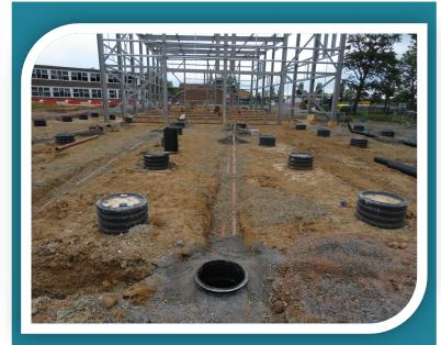
The foul drainage is installed using plastic pipe and connectors. These pipe runs are bedded on granular material to the designed falls. Each individual run will discharge into an 'inspection chamber' or 'manhole'.
