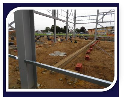
The sports hall floor construction is a block & beam system that sits on sleeper walls. These sleeper walls are built out of brick and blockwork.
