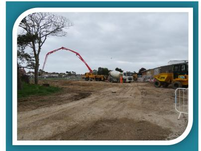
To install concrete into pads located in difficult positions we require the use of a concrete pump. This pumps the concrete into the already prepared excavation.
