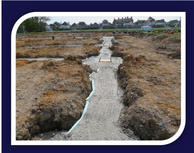
The filled excavations are levelled and bolts are positioned in accordance with the foundation drawing.
